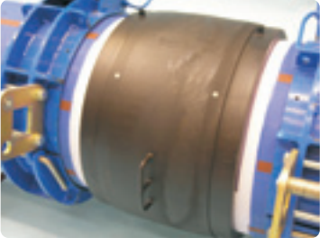
The second pipe is prepared and pushed onto the coupler
