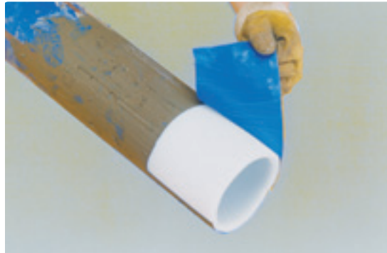
The natural core of the ProFuse pipe is protected by the sacrificial skin. The pipe is ready to joint without further preparation
